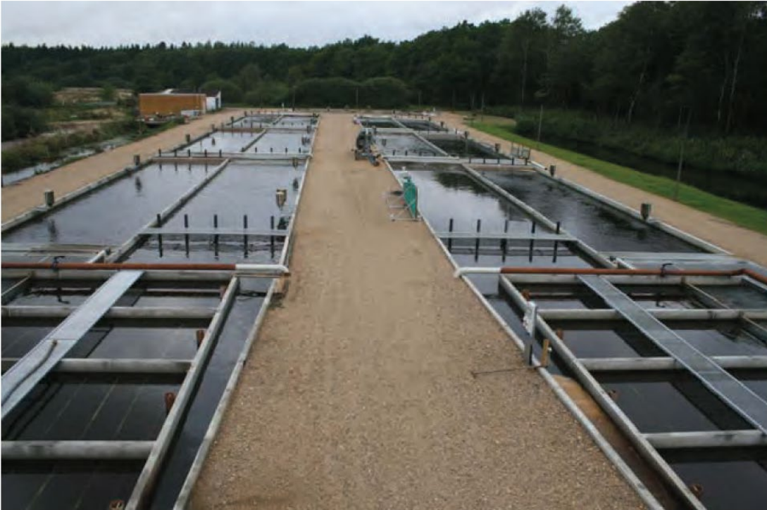
Model 3 – biofilter- Raibow trout production Denmark
