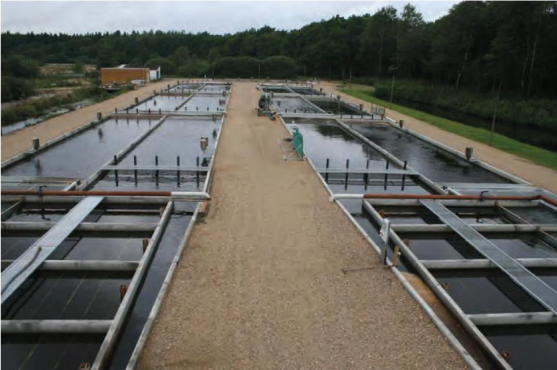
Model 3 – biofilter- Raibow trout production Denmark
